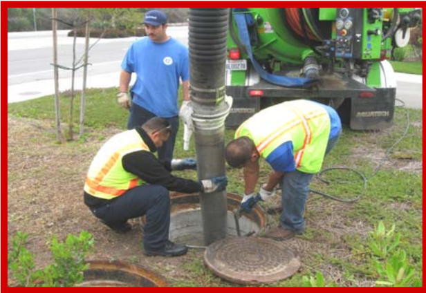
Remove Access Hatches Set Up Vacuum Truck to Clean The Pretreatment Chamber.
