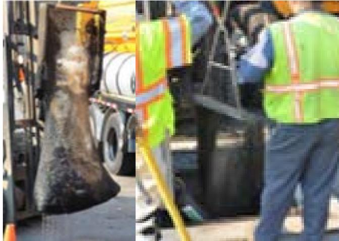
For sediment removal, the SiteSaver is designed with clear access at both the inlet and outlet. A vacuum truck, or similar trailer mounted equipment, can be used to remove the sediment, hydrocarbons, and water within the unit. For more effective removal, it is recommended to use sewer jetting equipment or a spray lance to force the sediment to the vacuum hose. When the floor is sufficiently cleaned, fill the system back to its normal water elevation (to the pipe inverts).
