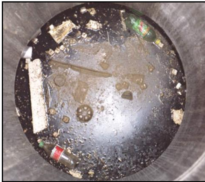
Floatable trash & debris in the Aqua-Swirl ®
