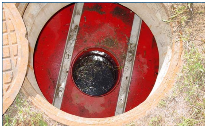
Figure 7: View over Center Shaft into sediment storage Zone
