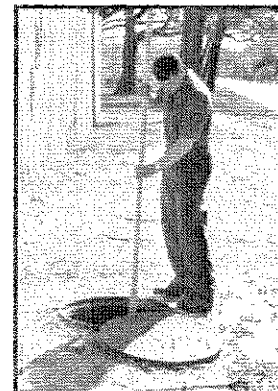
Sediment inspection using a stadia rod
