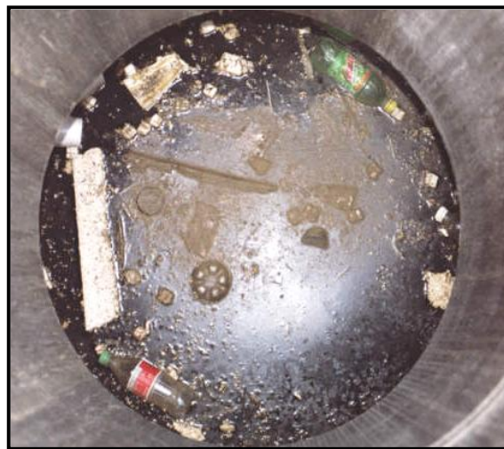
Floatable debris in the Aqua-Swirl ®
